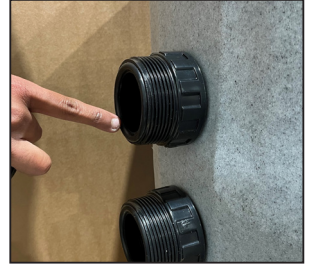
Take note that there is an O-Ring located inside the thread. Ensure this does not move during assembly.
